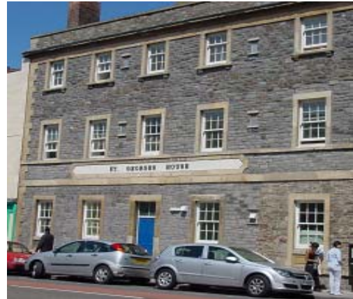
St George's House (Priority Youth Housing): Alternative to B&B for Young People
